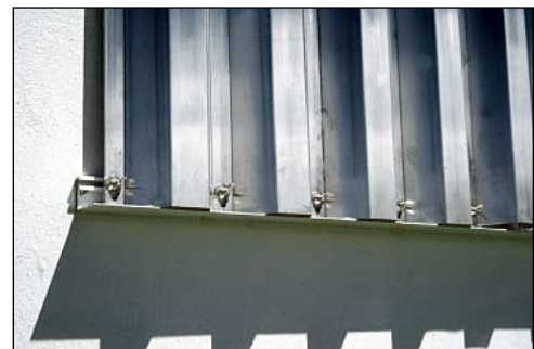
Figure 4. This metal shutter has top and bottom tracks that are permanently anchored to the wall (FEMA 577).
