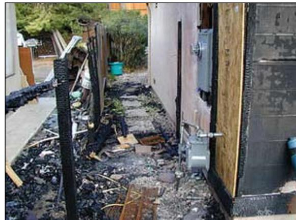
**Figure 1.** The gate that was attached to the garage at the corner ignited and led the fire to the home, causing the damage seen here ([firecenter.berkeley.edu](http://firecenter.berkeley.edu)).
