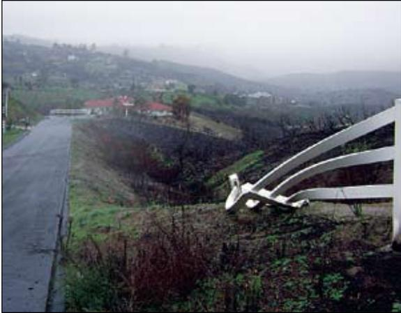
**Figure 2.** Plastic fences can melt even under moderate wildfire temperatures (FEMA field team).
