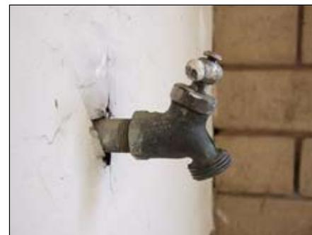
**Figure 1.** The gap around utility penetrations such as this one should be filled.
