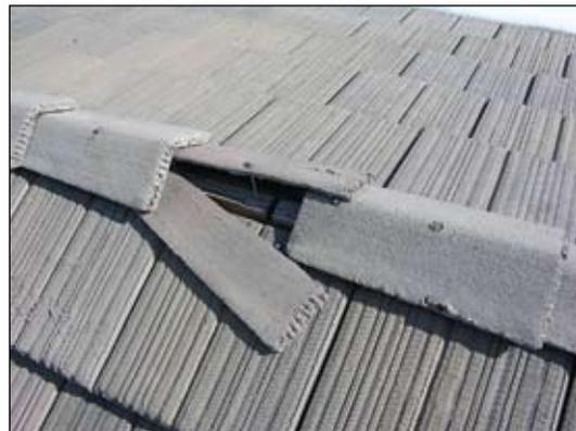
**Figure 3.** Displaced tiles allow ember entry.
